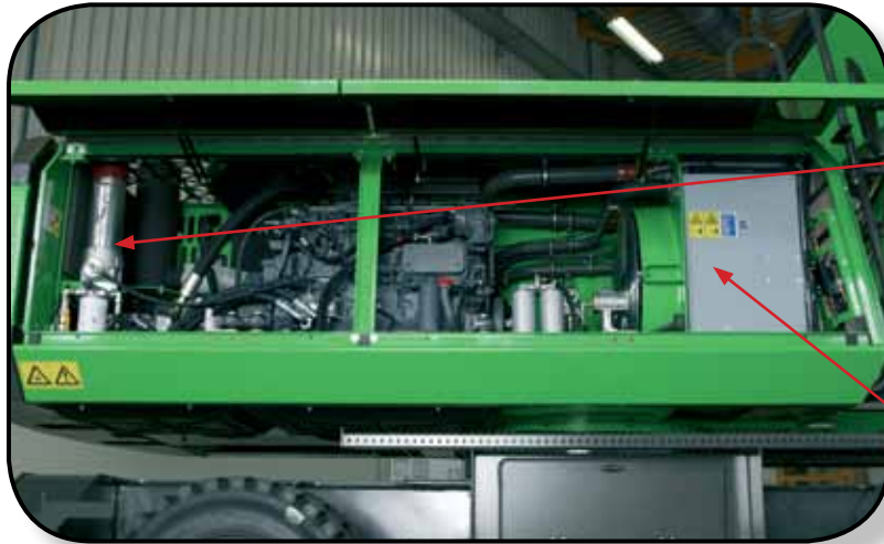
Ideal maintenance access from ground level.
